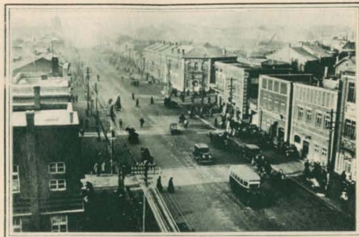
RAILWAY ZONE, HSINKING
